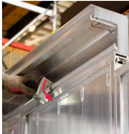
Swivel in the Space Coupler from above - the wedge is always on the left.
