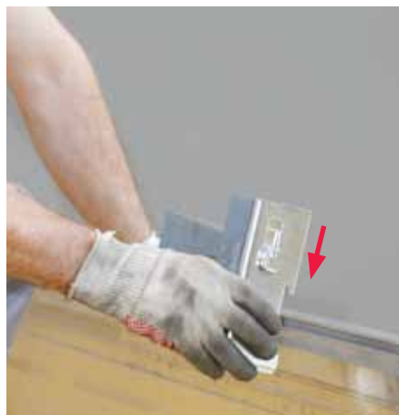
Connect the External Corner Profile and Wall Panel with Wall Couplers.
