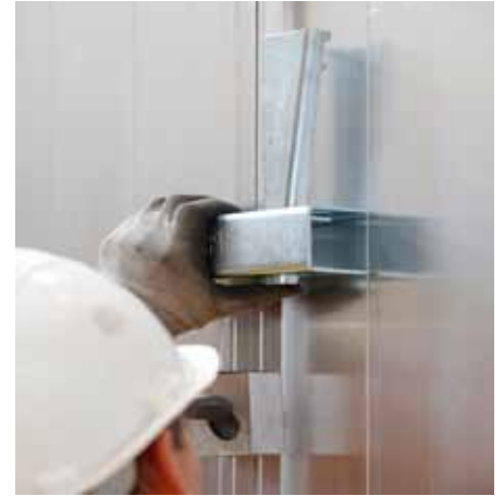
Place Wall Coupler on the Edge Profile with one hand.
