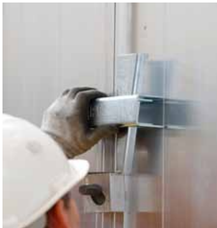
Loosen wedge - wedge falls to a middle position.
