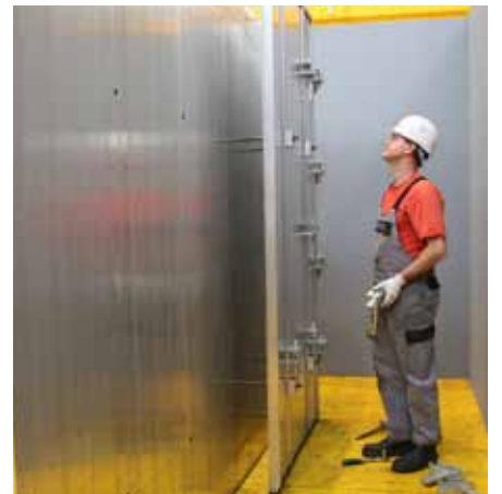
Connect Panels with Wall Couplers. Tighten anchors.
