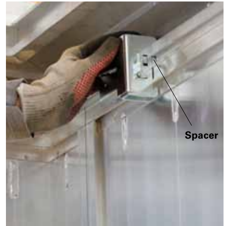
The Space Coupler must be securely positioned in the joint.
