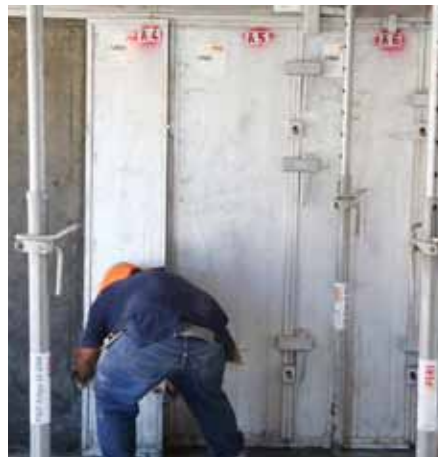
Dismantle the panels - remove from concrete from bottom to top.
