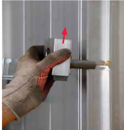
Place Anchor Sleeve together with the locking slide which has been pushed upwards in the tie hole.
