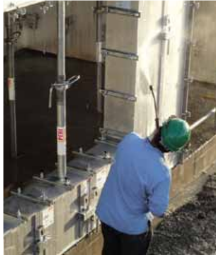
Clean panels with water immediately after concreting, e.g. high-pressure hose.
