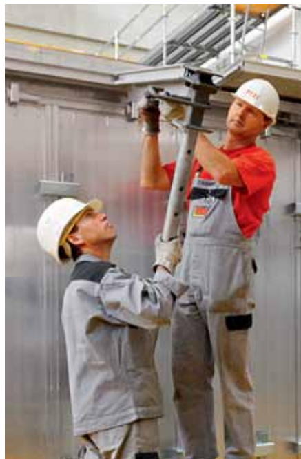
Mount slab prop with drop head in the slab beam from below.
