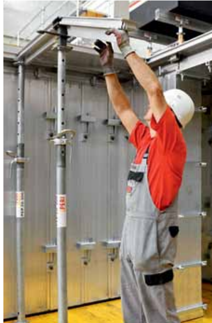
Mount Slab Beam.
