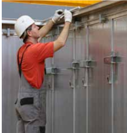
Level the position of the Slab Beam.
