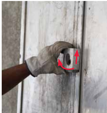
Remove Anchor Sleeve - push up locking slide and dismantle by twisting to one side.
