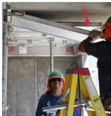
Strike further Slab Panels.
