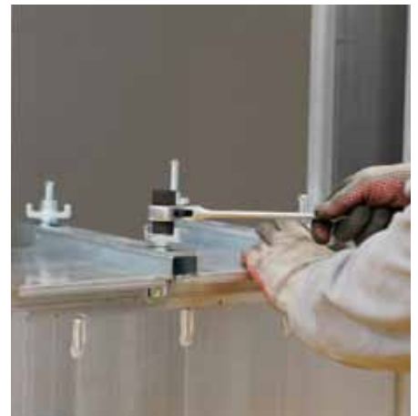
Firmly tighten nut with a spanner.
