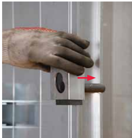
Place Anchor Sleeve together with the locking slide which has been pushed upwards in the tie hole.
