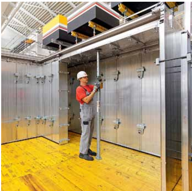
If necessary, position push-pull props, see plan.
