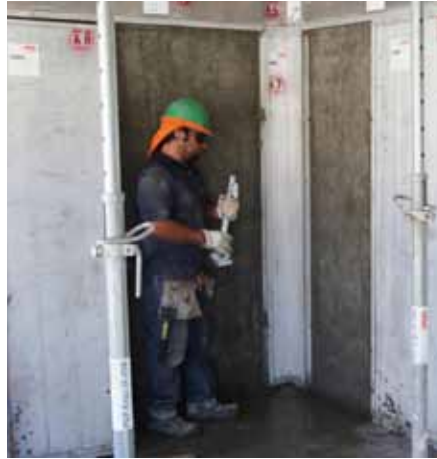
Striking with Striking Tool W/S.
