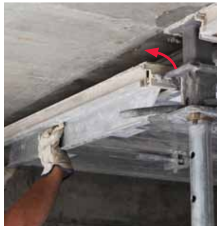
Remove Slab Beam.
