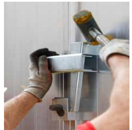
Lightly hammer in wedge with a rubber or plastic hammer.
