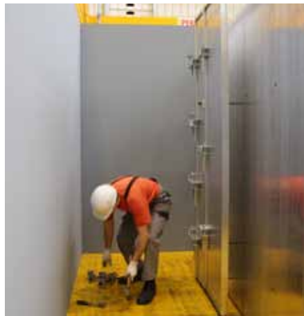
Connect using Wall Couplers.
