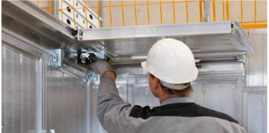
Position Slab Panel without Slab Beam. Secure with one slab coupler per panel side.
