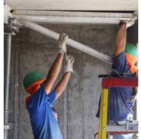
Remove final Slab Panel in the row.
