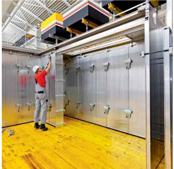
Connect side formwork and Wall Panel with wall, slab and screw couplers, see plan.
