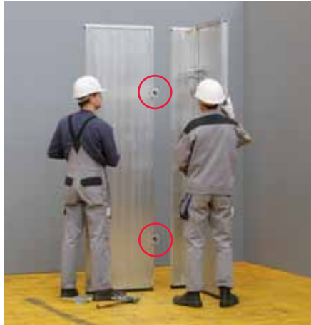
Insert the Anchor Sleeve on the right-hand side of the next panel and secure.
