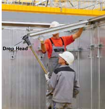
Mount the Slab Prop with Drop Head in the Beam Head, see B8.
