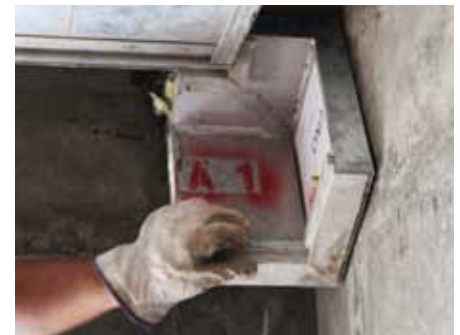
Pull out Transition Corner from below.
