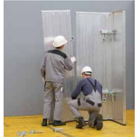
Position Wall Panel.
