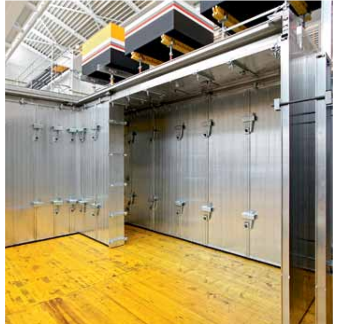
The beam formwork is now assembled.
