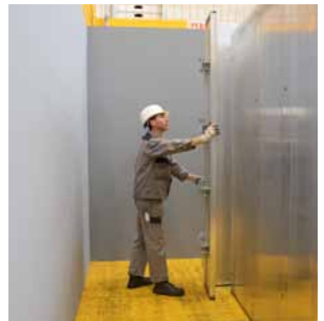
Position External Corner.
