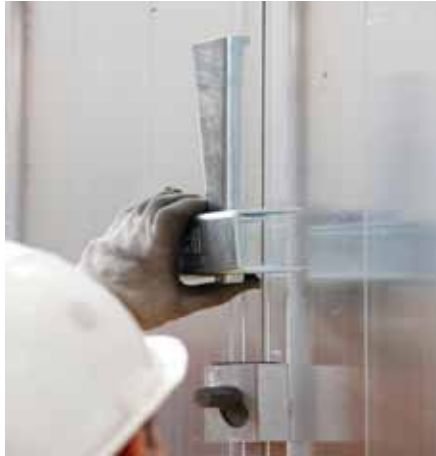
Place wedge in upper end position.
