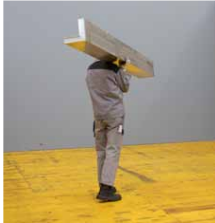
Position the Internal Corner Panel.
