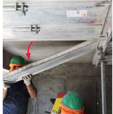
Slab Panel is folded downwards.
