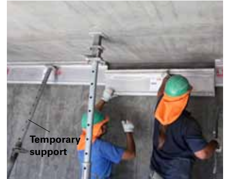
Position temporary support.
