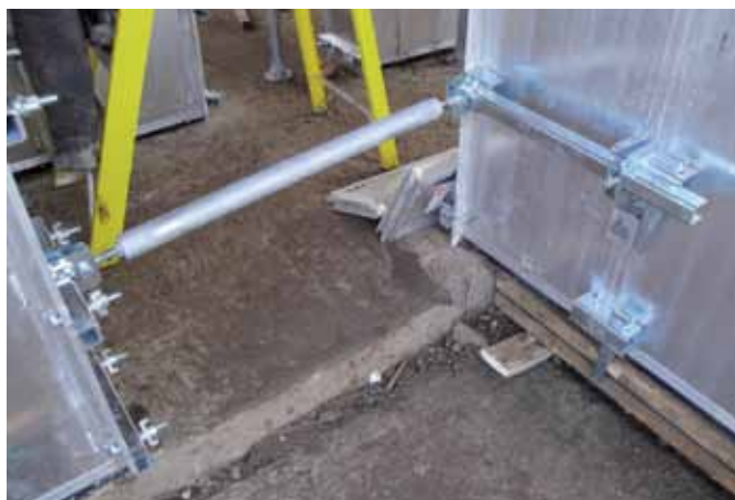
Right-angled wall sections
