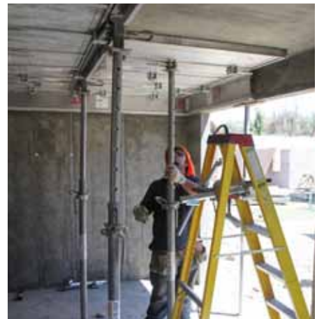
Re-position temporary support.
