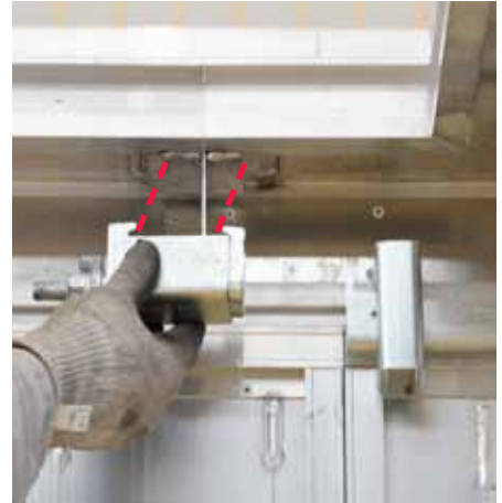
Push Screw Coupler over the Flange Profile.
