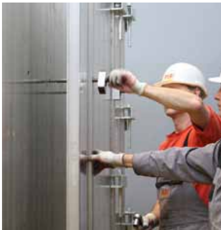
Install anchors.
