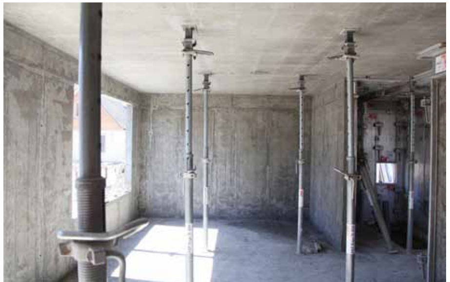
Striking of the room is now completed.
