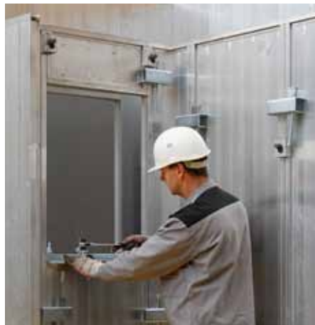
Fix bottom formwork by means of Stop End Walers.
