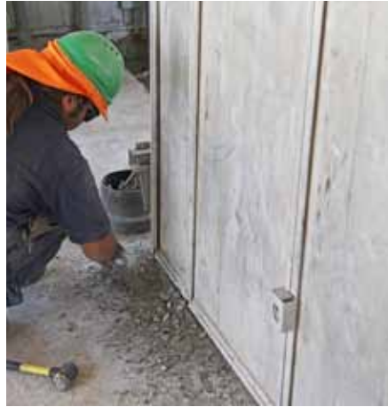
Remove concrete residue.
