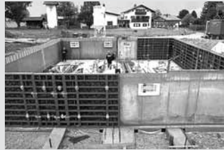
Wall Formwork
