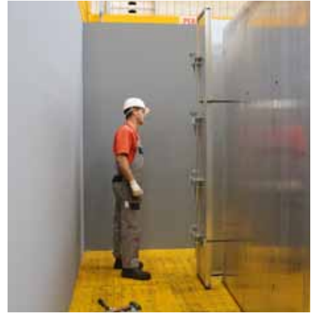
Install ties on one side - above.
