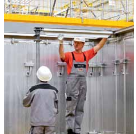
Swivel up the Slab Beam and align.
