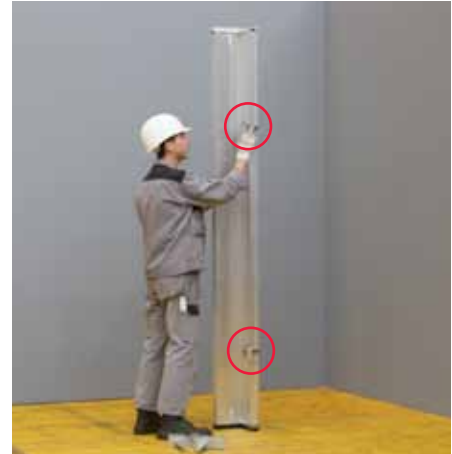
Insert the Anchor Sleeve on the right-hand side of the panel and secure, see A6.
