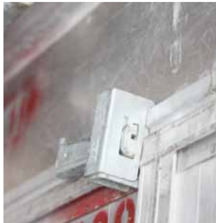
Remove Anchor Sleeve - push up locking slide and dismantle by twisting to one side.
