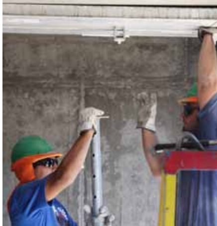
Support the final Slab Panel by hand. Remove temporary supports.
