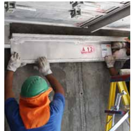
Remove Transition Panel.
