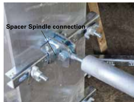
The Spacer Spindle connection is firmly connected to the Stop End Waler.
