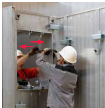
Side formwork is positioned between the bottom formwork and soffit formwork- this needs to be supported.
