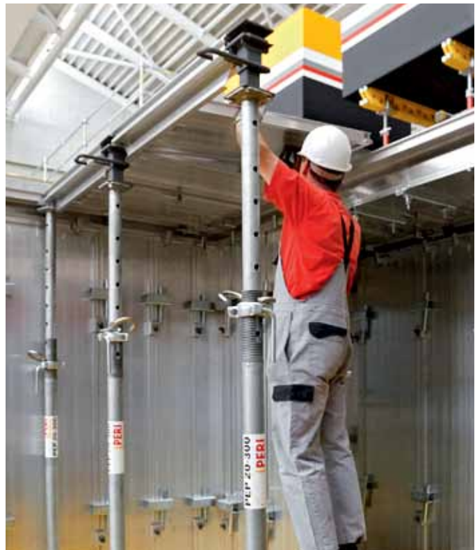
Mount Slab Panel and secure with Slab Couplers.
