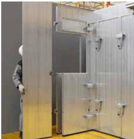
Position Wall Panels next to the opening and connect by means of Wall Couplers.
