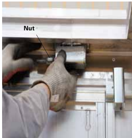
Screw on nut by hand.
