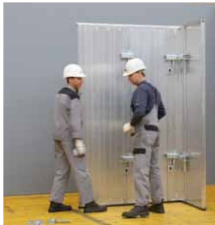
Connect Panels with Wall Couplers. Take height adjustments into consideration.
