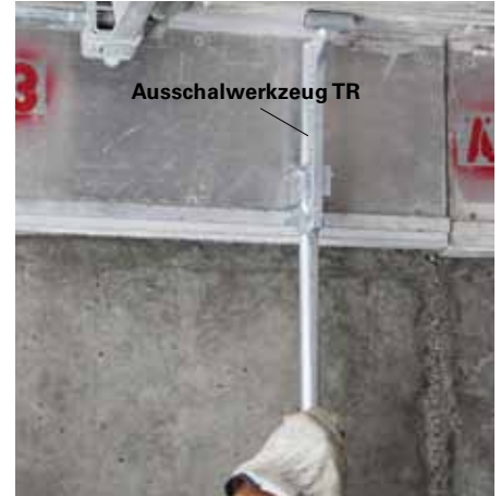
Release Transition Panel from the concrete by means of Striking Tool TR.
