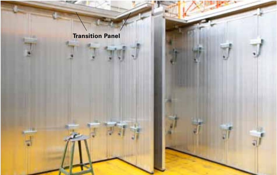
Continuously install Transition Panels.
