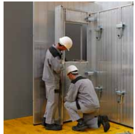
Lift Internal Lintel Panel and secure with Wall Couplers.
