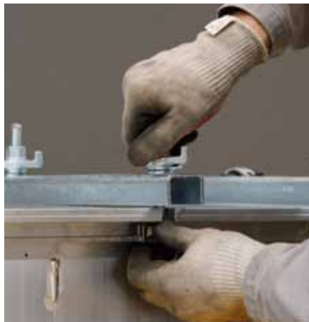
Tighten nuts by hand.
