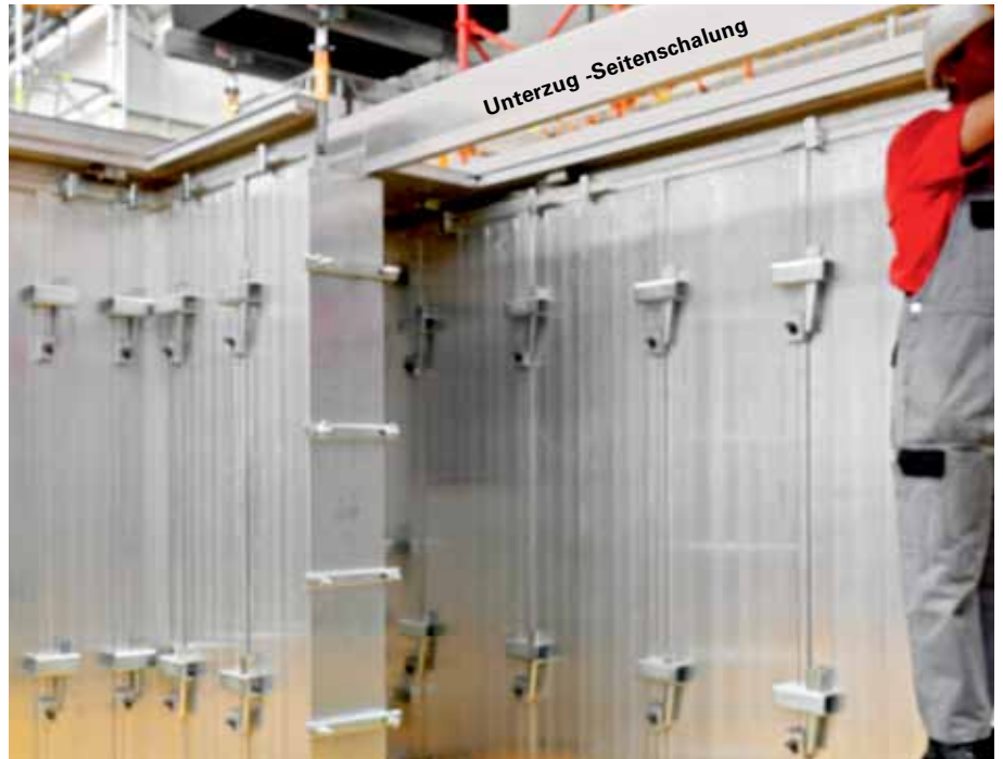
Install side formwork for the beam.
