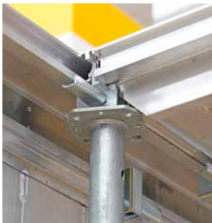
Support with slab props.
