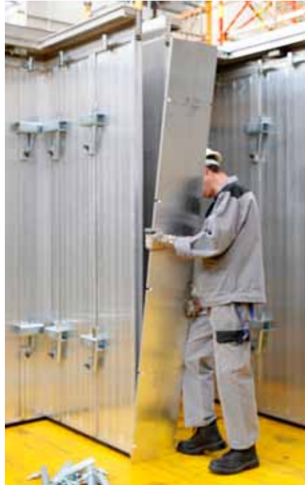
Starting from below, push Stop End Profile onto the front end of the Wall Panel. Check the wall thickness.
