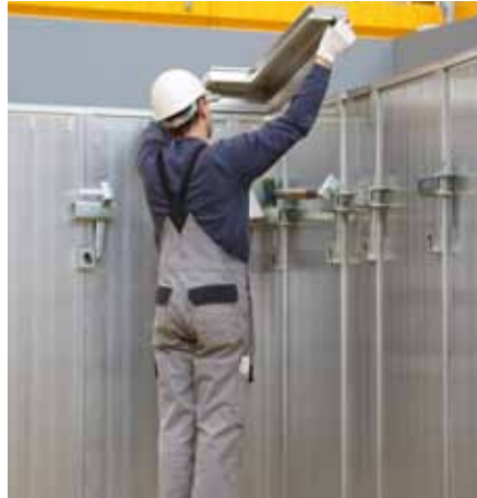
Begin in the corner with the Transition Panel with Corner Piece.
