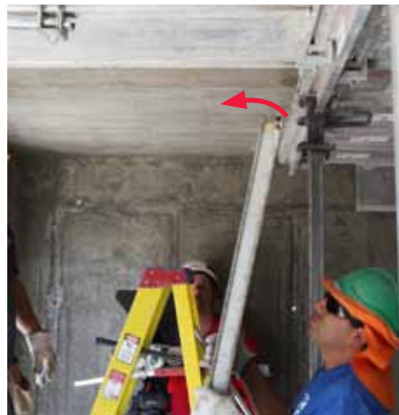
Remove Slab Panel.
