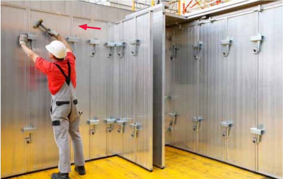
Shutter additional Wall Panels.
