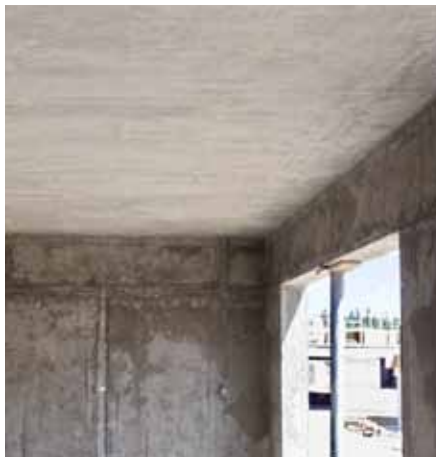
Striking of the slab area is now complete.
