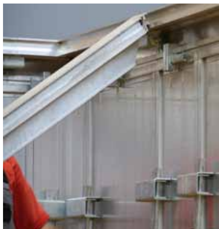
Mount the Slab Beam in the Transition Panel.
