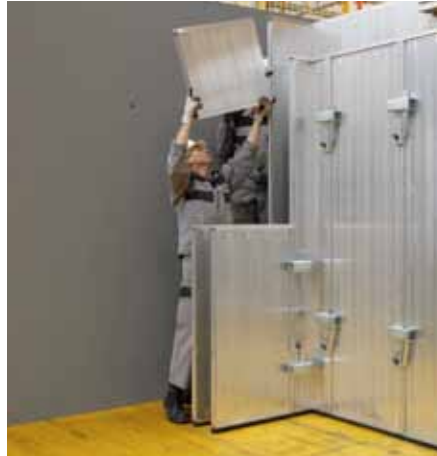
Mount Screw Coupler on the External Lintel Panel. Lift the External Lintel Panel.
