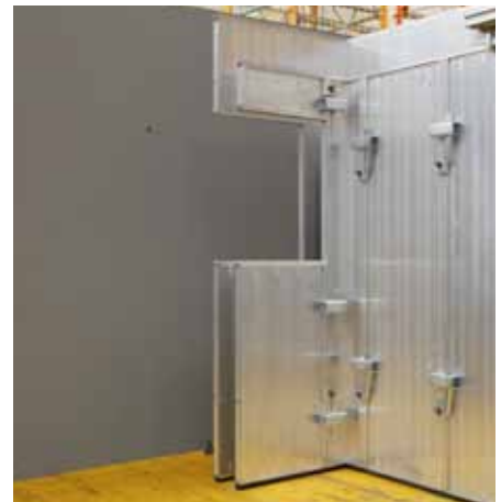
Lift Internal Lintel Panel and secure with Wall Couplers.
