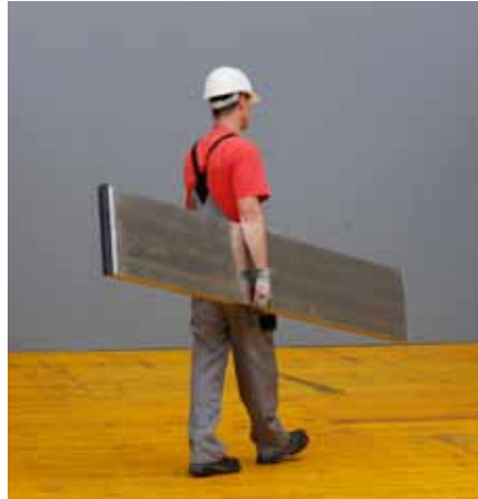
Position first Wall Panel of the external corner.
