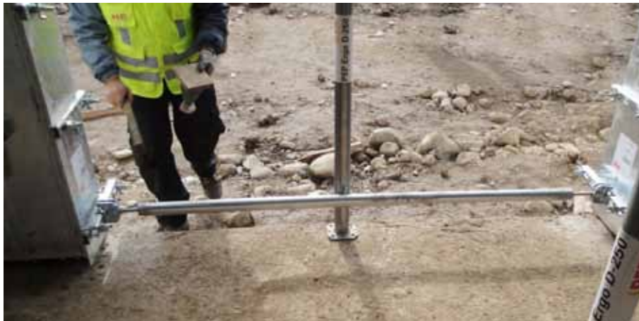
Parallel wall sections
