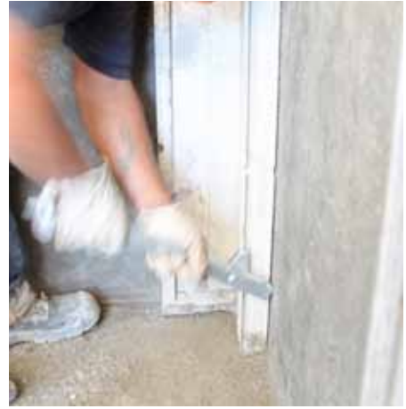
Attach Striking Tool W/S with the claw in the Edge Profile.
