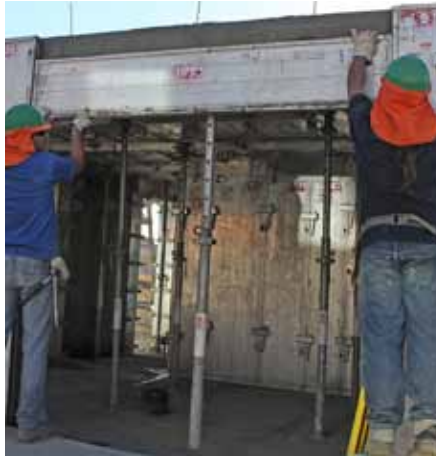
Remove External Panels on the openings.
