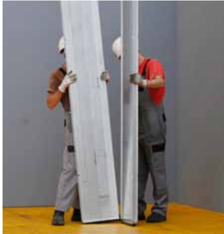
Push second Wall Panel into the External Corner Profile and connect by means of Wall Couplers.
