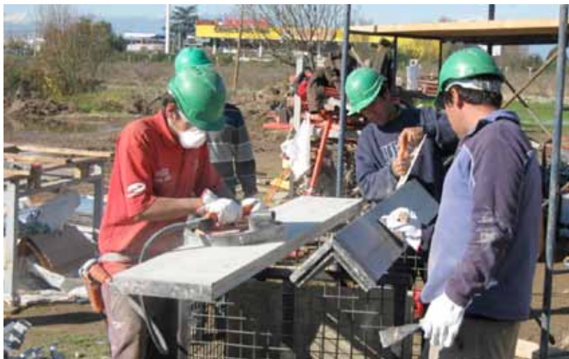
Clean panels after every use, eg. with rotating brushes.
