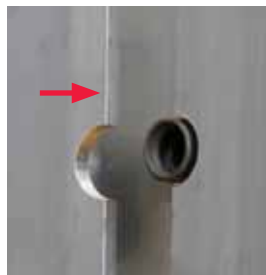
Push the next Wall Panel with the semi-circular cut-outs over the Anchor Sleeve.
