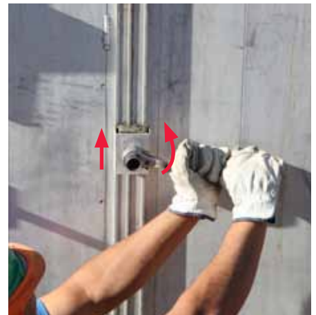
Loosen ties with a quarter turn and push locking slide upwards.
