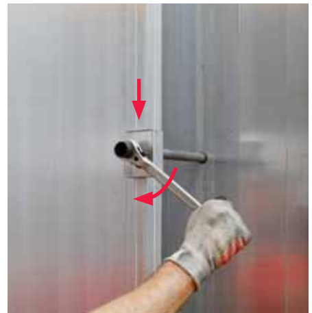
Push locking slide downwards. Tighten anchor with wrench or ratchet.
