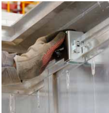
Swivel in the Space Coupler from above - the wedge is always on the left.
