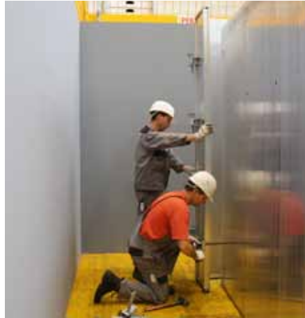
Install ties on one side - below.
