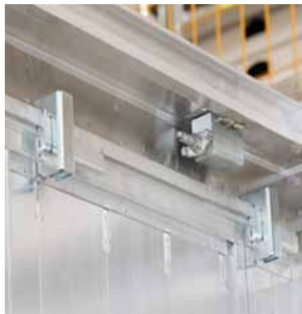
The Screw Coupler is now installed.
