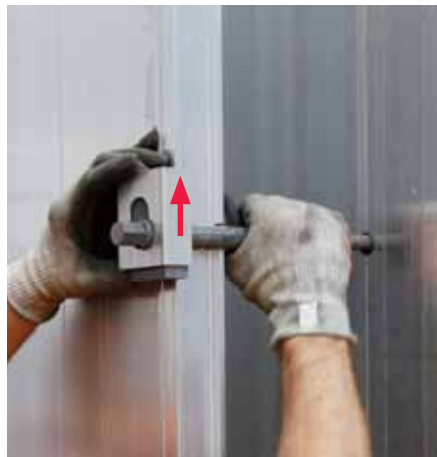
Hold locking slide in the top position. Screw in anchor by hand.
