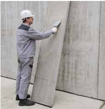
Clean the panels immediately after striking, e.g. with a spatula.
