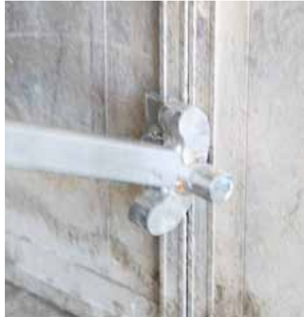
Attach Striking Tool W/S with the claw in the Edge Profile.
