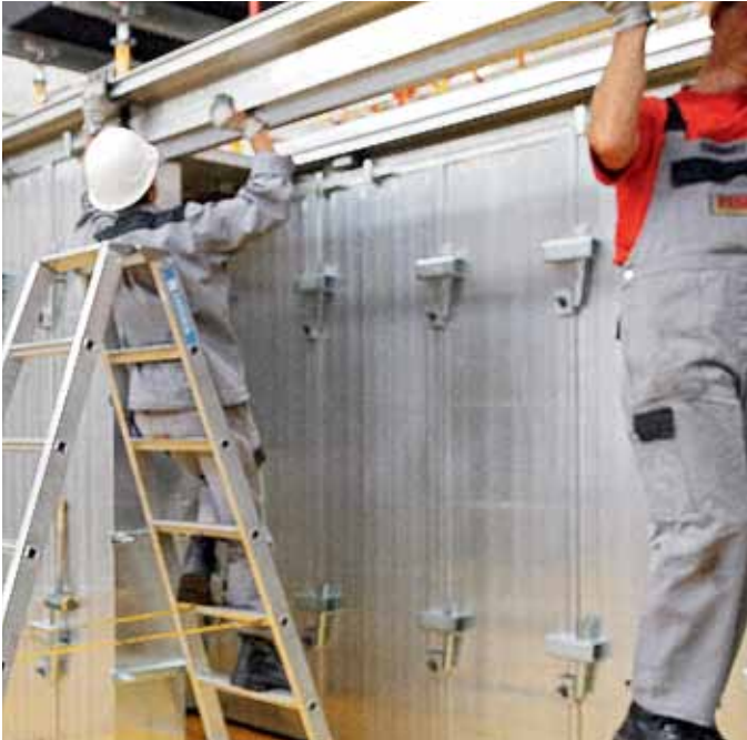
Lift second set of side formwork for the beam.
