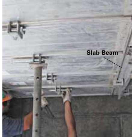
Secure the free end of the Slab Panel with one hand. Remove Slab Coupler on adjacent panel.
