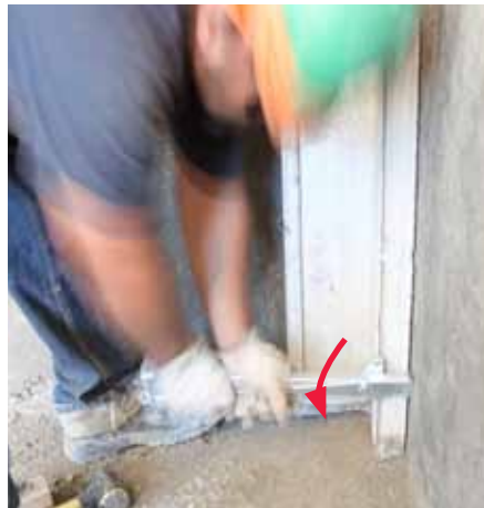
Push Striking Tool W/S upwards or downwards until the panel is released from the concrete.
