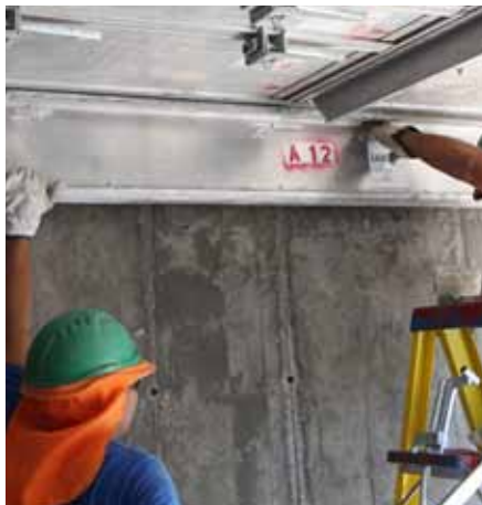
Turn bottom longitudinal side away from the concrete.
