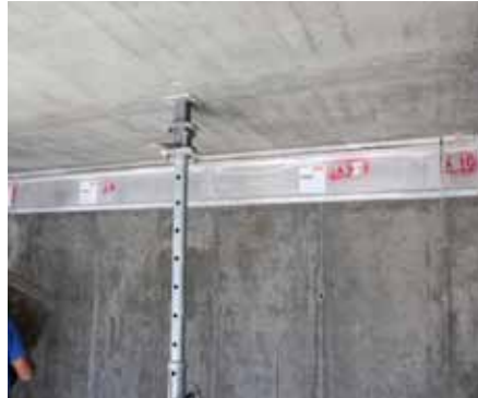
Remove final Transition Panel.
