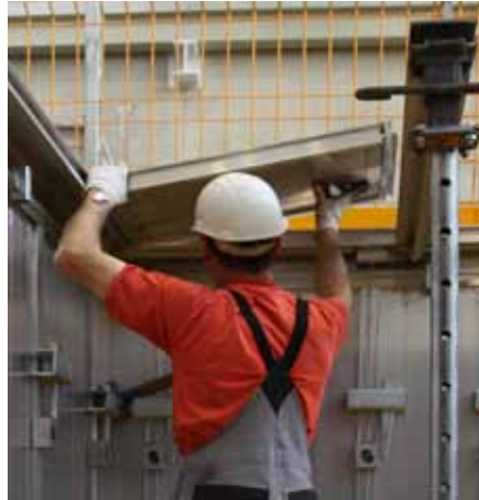
Place Slab Panel between the Transition Panel and Slab Beam.
