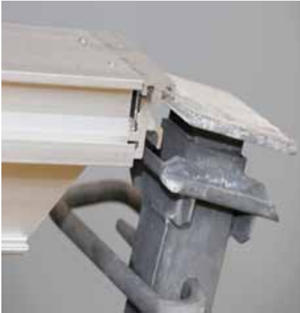
Align Drop Head in the beam axis.
