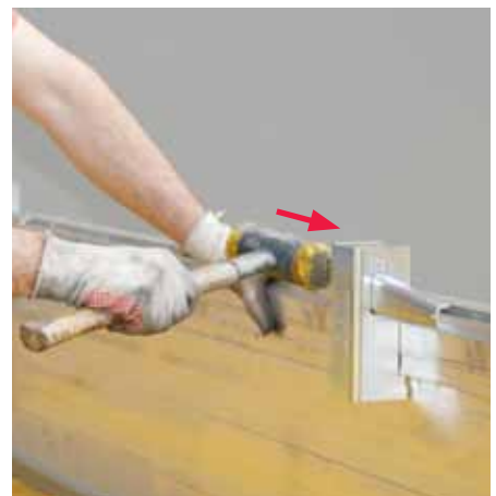
Hammer in wedge tightly.
