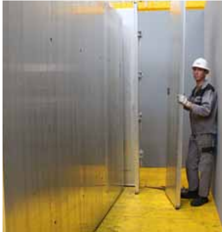
Prepare Wall Panel for installation.
