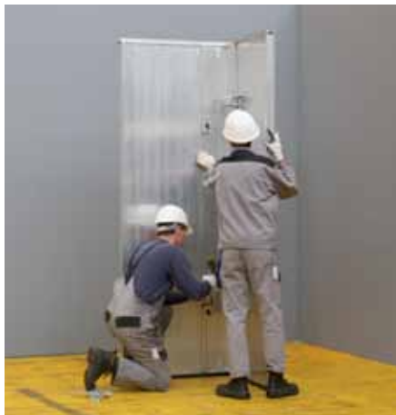
Connect the Wall Panel and Corner Panel with Wall Couplers - see plan for number of couplers used. The internal corner area is now assembled and is in position.
