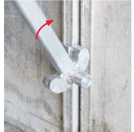
Push Striking Tool W/S upwards or downwards until the panel is released from the concrete.
