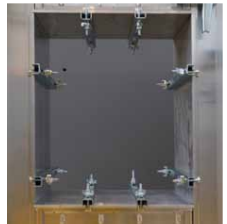
The stopend formwork for the opening is now ready.
