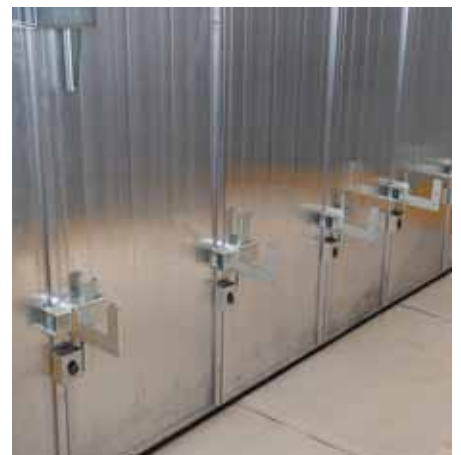
Install Alignment Couplers on every panel joint. Secure in the same way as a Wall Coupler.
