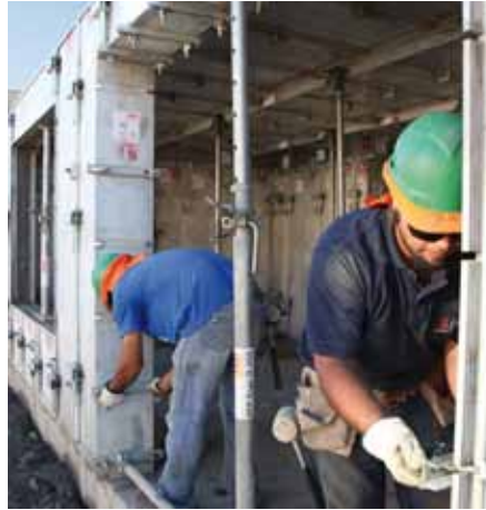
Remove all Stop End Profiles.
