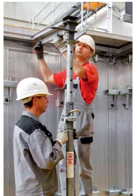
Place slab prop in a perpendicular position and spindle out to reach the required height until the slab beam is horizontal (spirit level).
