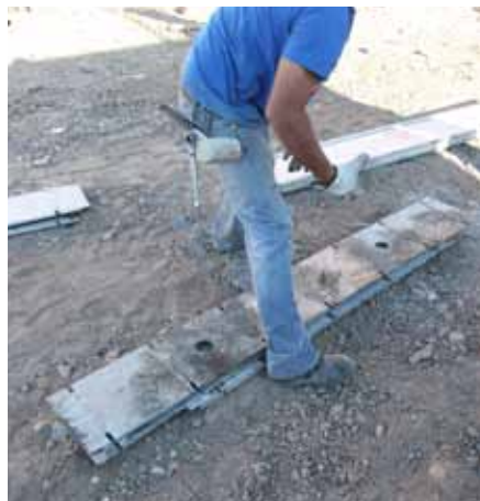
Dismantle the Stop End Profiles on the beam - quickly remove slab props. Static proof provided by contractor.
