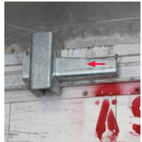
Remove Spacer Couplers. Hammer wedge to the left.
