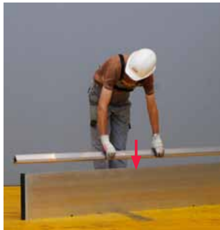
Place External Corner Profile in the Edge Profile of the Wall Panel.
