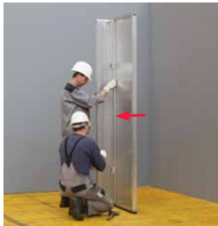
Push the next Wall Panel with the semi-circular cut-outs over the Anchor Sleeve.
