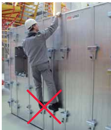
Formwork couplers and ties are not to be used as climbing aids!
