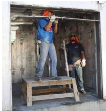
Dismantle the Stop End Profiles on the beam - quickly remove slab props. Static proof provided by contractor.
