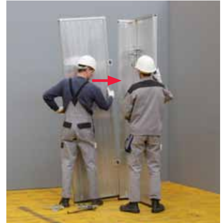
Push the Wall Panel with the Anchor Sleeves in the semi-circular cut-outs of the Corner Panel. Carry out any necessary height adjustments.
