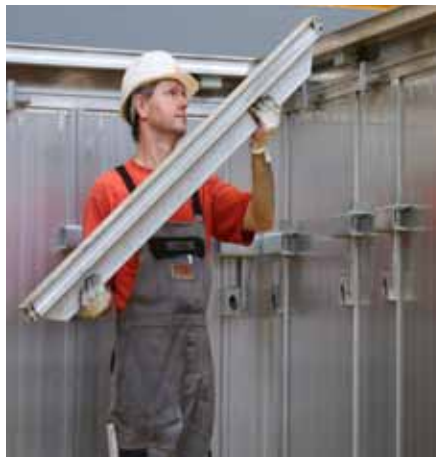
Mount the Slab Beam in the Transition Panel.
