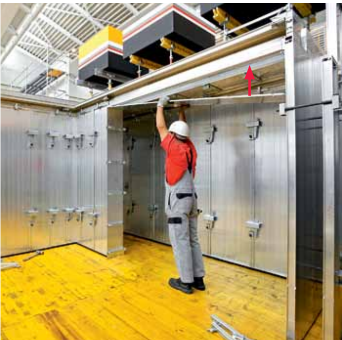
Lift soffit formwork for the beam (Stop End Profile).
