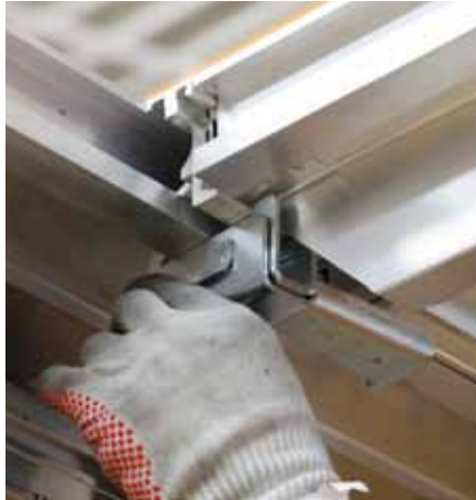
Connect Slab Beam to the Transition Panel with Slab Couplers.
