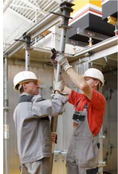
Mount slab prop with drop head in the Slab Beam from below and swivel upwards.
