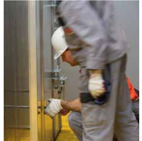
Install anchors.
