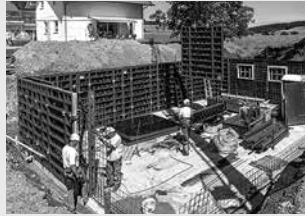
Wall Formwork
