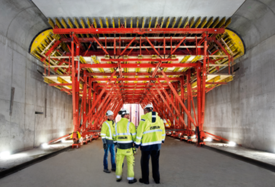
Marieholm Tunnel, Gothenburg, Sweden Züblin Scandinavia AB
